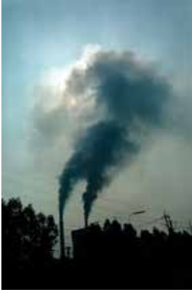
IP Power Station
